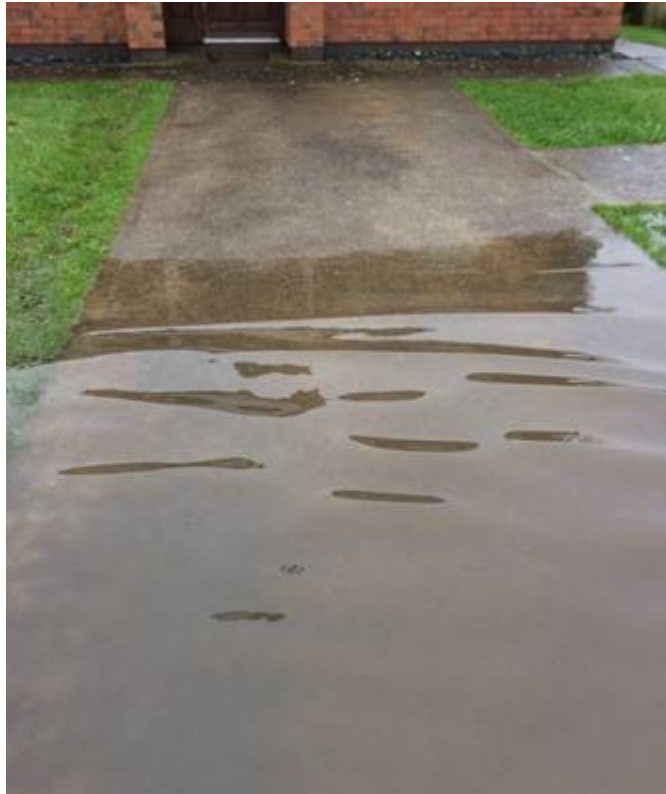
Figure 3 : Worst Affected Property from Surface Water Flooding – Lakeside Crescent
